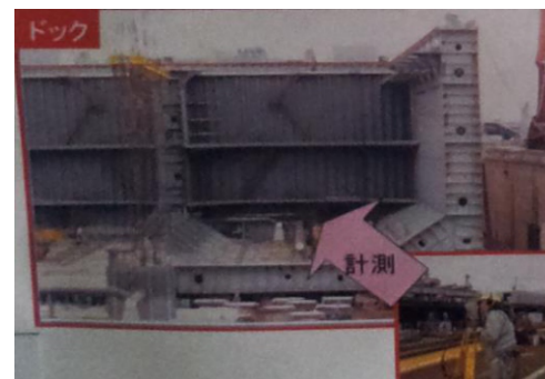
<Measuring for Erection>
